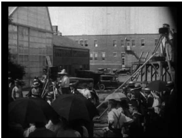
Figure 3. Outside the Paragon complex with one of the sliding glass panels from the main building folded upwards
